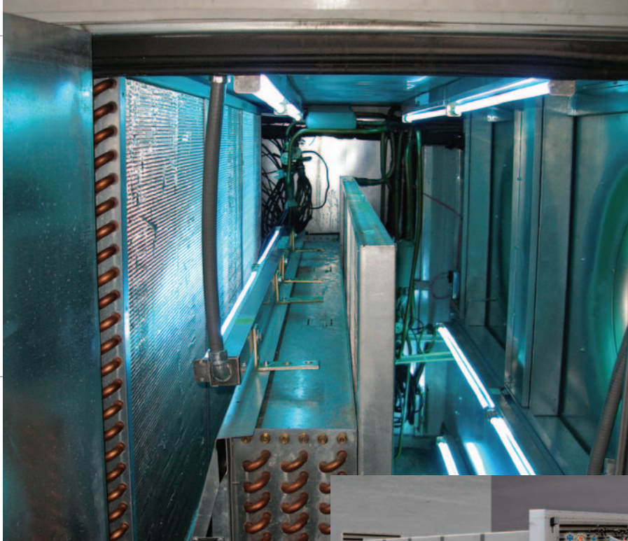
Anatomy of UVC: (clockwise) A large commercial A/C unit featuring UVC lighting; visual inspection is recommended for checking UVC systems, but not for making changeout decisions; an air-handling-system schematic shows proper location of UVC lamps at the downstream side of the cooling coil.
