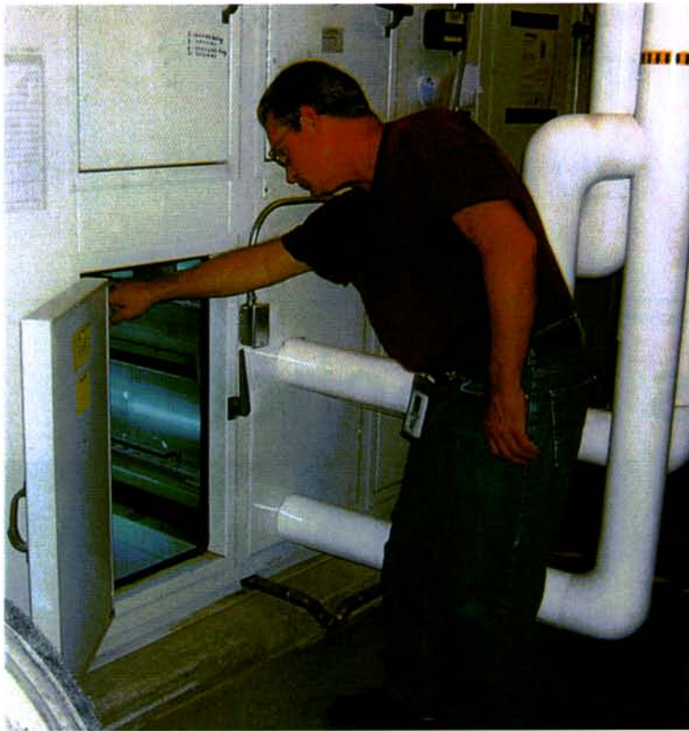
Ron Bjorklund, district-wide maintenance at Robbinsdale (Minn.) Area School District 281, inspects one of the air-handling units. The school installed UVC lights to help prevent mold growth.
