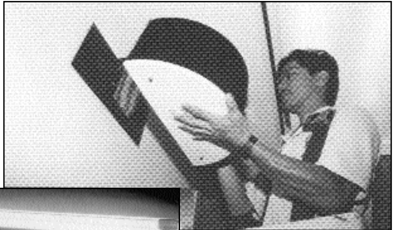
The Queen's Medical Center in Honolulu has installed upper-air UVGI fixtures for individual room disinfection (above) and in air-handling units (left) to improve air quality, protect against surface mold and bacteria, kill or inactivate airborne pathogens, and maintain energy efficiency.
