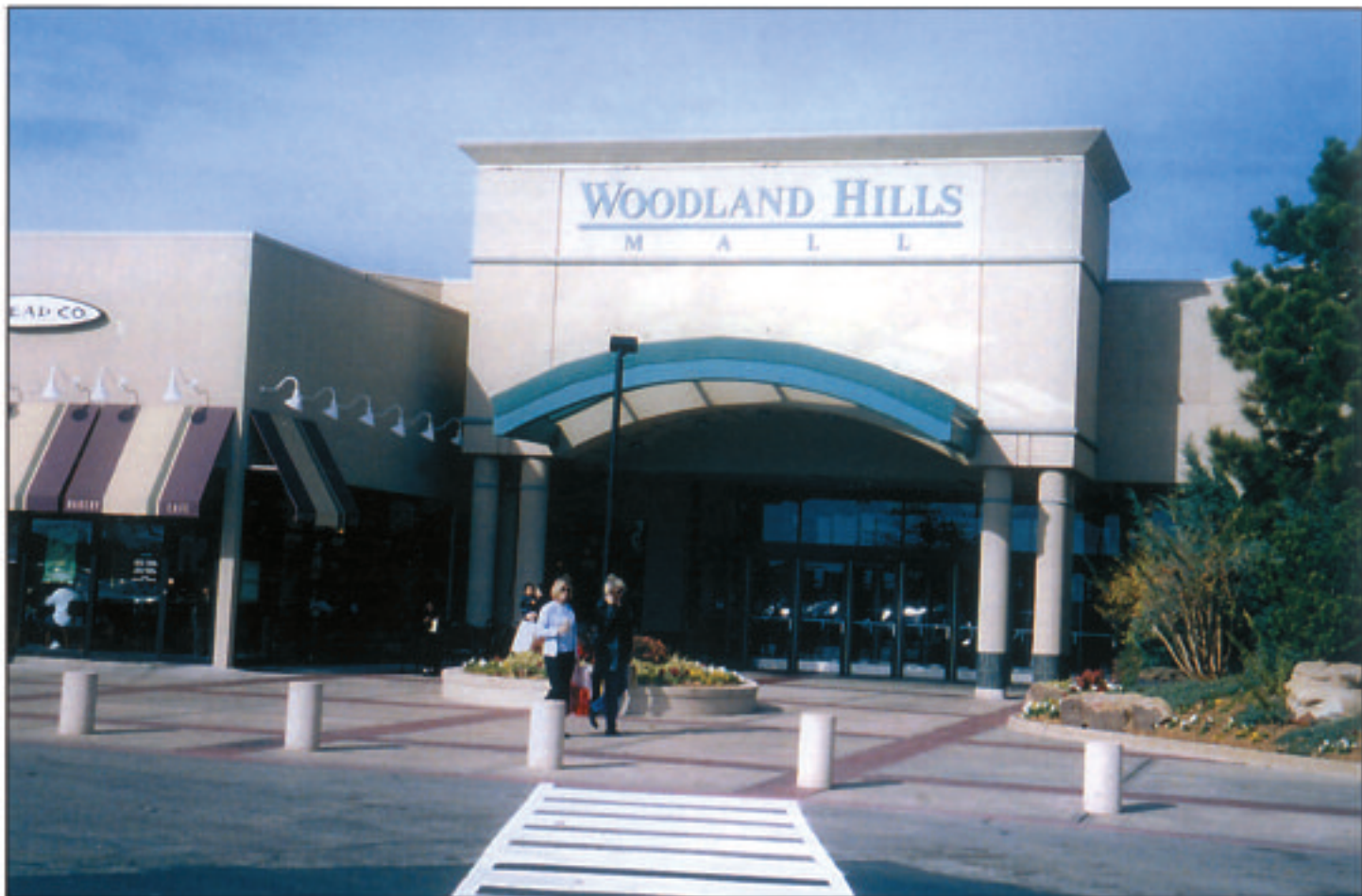
Woodland Hills Mall was built in 1975, then underwent an expansion that was finished in 1982. An extensive HVAC retrofit of the 165-store, 1.1-million-sq-ft complex was completed in September 2000.
